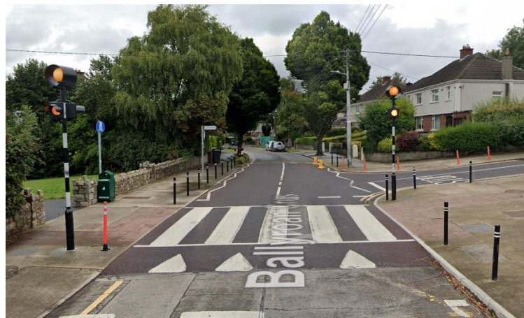
Figure 2 Newly upgraded Zebra Crossing in DLRCC – Mains powered with raised platform
